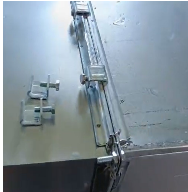
Figure 16. Rectangular duct transverse flange joints sealed with corner clamps and EPDM gasket
