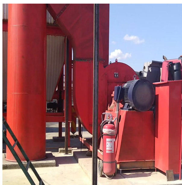
Figure 3. Dust extraction fan serving the asphalt production plant [20]
