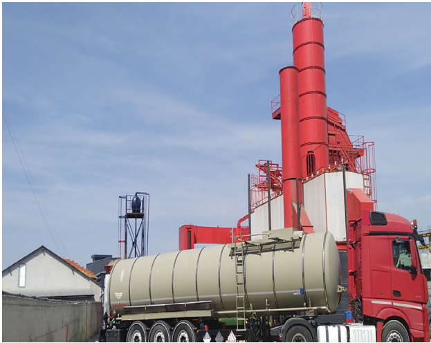
Figure 4. Dust exhaust ductwork of the production facility
