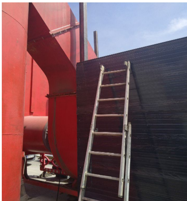
Figure 8. Acoustic enclosure installed over the main drive motor of the asphalt station
