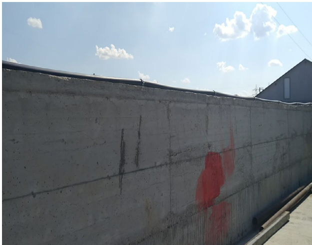
Figure 11. High-pressure (10 bar) perimeter mist curtain system mounted on the boundary wall
